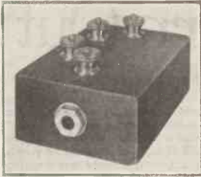
C. F. Ewcell, Ltd. Fig. 4.—Enclosed Jack.
