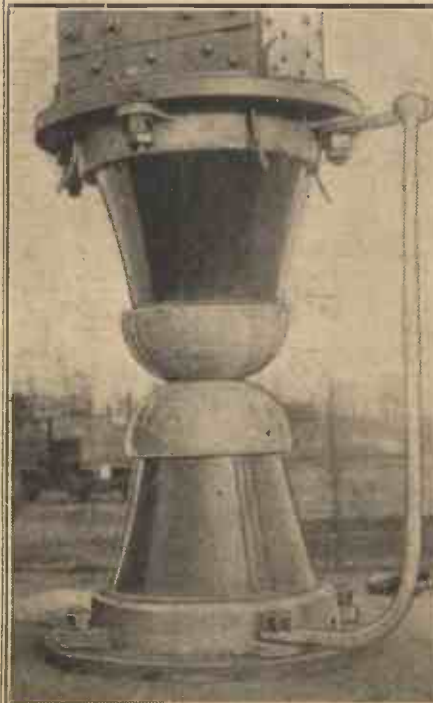
This is the base of Budapest's new aerial mast, one of the highest structures in Europe. The whole weight is taken by the porcelain blocks, the rod to the right being merely for earthing the metal structure.
