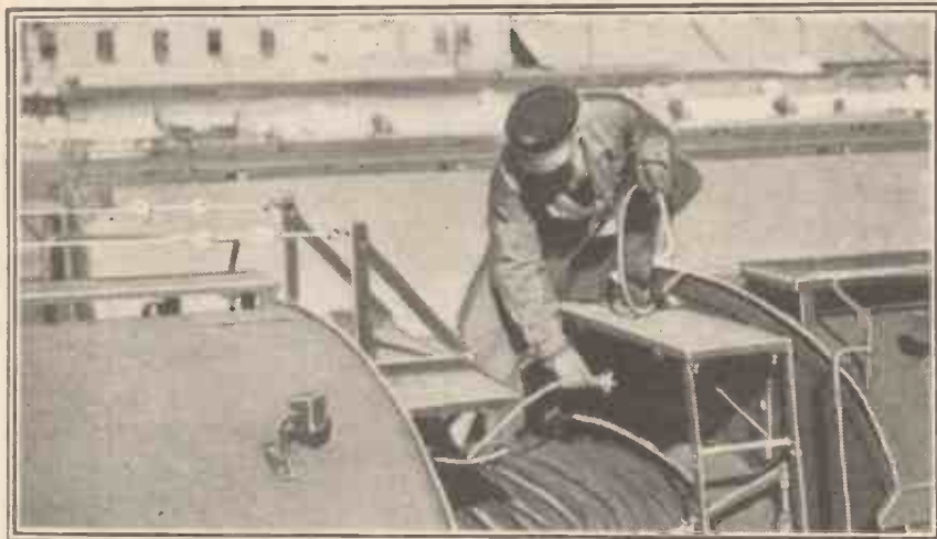
Many trains in Germany are equipped with radio receivers for entertaining the passengers. This photograph shows an engineer linking up a couple of carriages.
