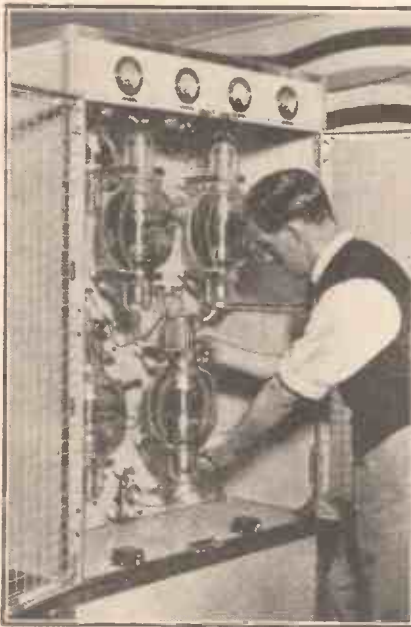
Putting the giant valves in the B.B.C. relay amplifier at Olympia. It fed about 400 loud speakers.
