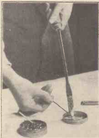
Tinning the wire before making a joint will save time and trouble in the long run.
