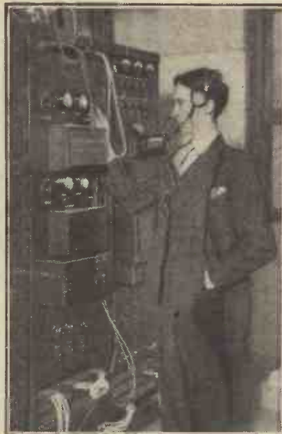
A section of the radio installation at the Pennsylvania Hotel, New York.
