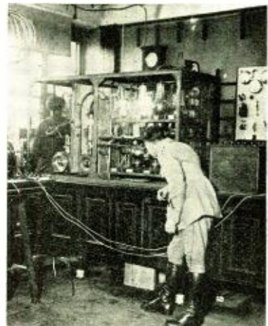
The Eiffel Tower radio broadcasting station in Paris. Here are the tubes
