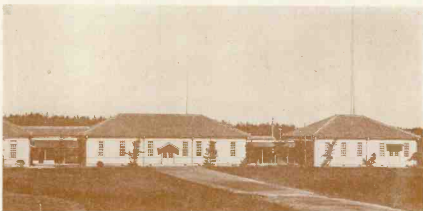
The receiving and control station at Tomioka
