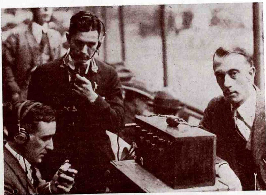
Input equipment installed at the Yankee Stadium with E. F. Grossman at left and A. W. Protzmann standing, who operated the input apparatus, and at right Graham McNamee, who described four of the games for WEA, WGY and WJAR
