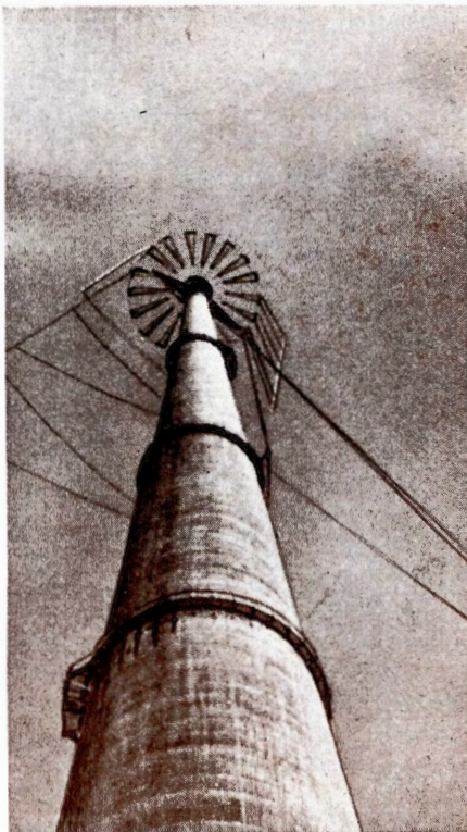
The 600-foot concrete mast of the transmitting section of the Iwaki plant at Haranomachi, which was not damaged. It is 55 feet in diameter at the base and four feet at the top
