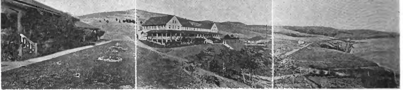
One of the things that makes a radio operator's life pleasant is a view such as this. The operators and engineers who make their homes at Marshall, Cal., have this prospect before their eyes. Cottages, hotel, power house, hills and sea all unite kindly and gently
