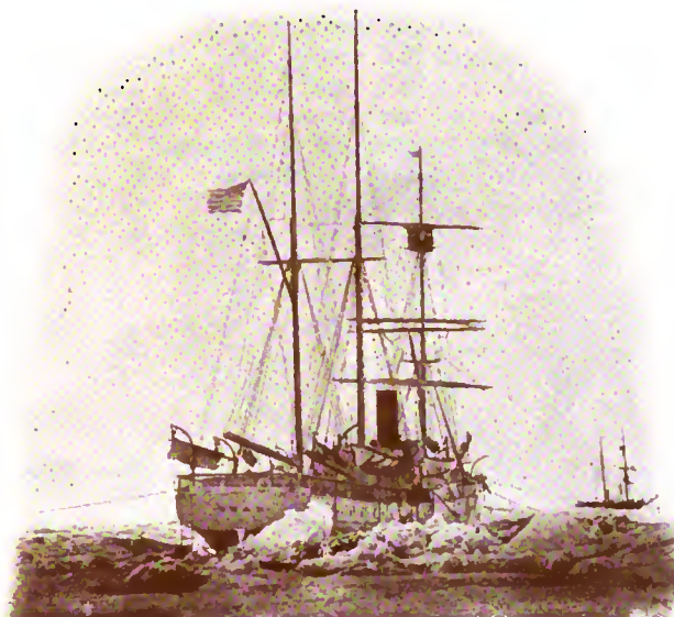
The "Bear" at its work amid the icy floes. Its masts are far higher than any sails could be carried—they support something more vital than sails—the radio antenna
