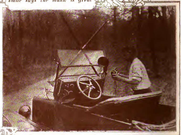
This fella is a wise young bird, for 'way last Spring (see the bare trees?) he had his automobile all fixed up like this, with receiver and loop mounted on the dash, and since then he has been seen on the highways and byways here and there, picking up local and DX programs
