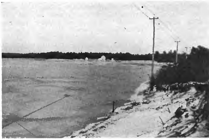
View of the nine-mile antenna at Riverhead, L. I., used for static reduction in trans-Atlantic reception by the Radio Corporation of America
