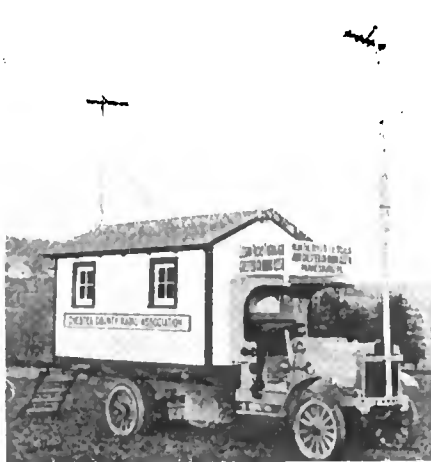
Chester County Radio Club's station installed in a motor bus
