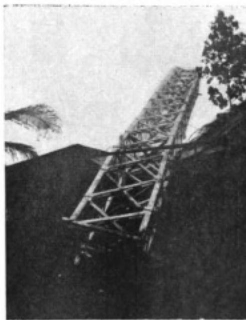
Where the tower went through the roof
