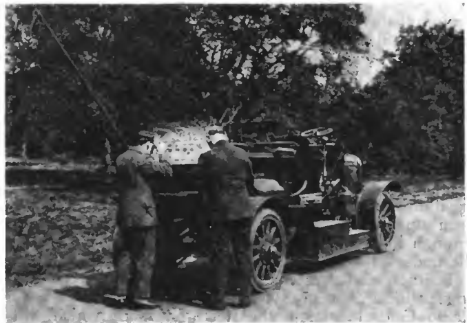
Underwood Firemen operating a wireless telephone installed on rear of fire tender
