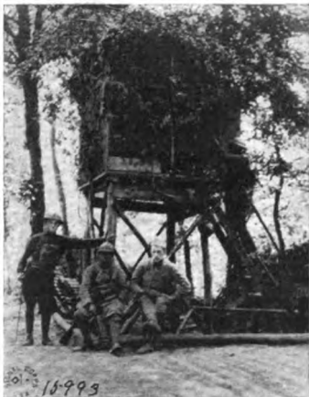
A signal station for visual communication captured from the Germans by American signalmen
