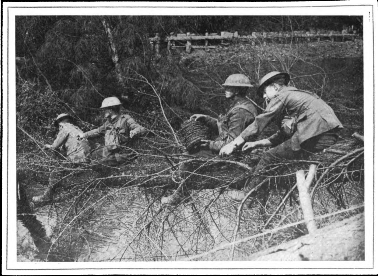
When trees were felled to block a canal their removal by the enemy was impeded by weaving the wire through the branches
