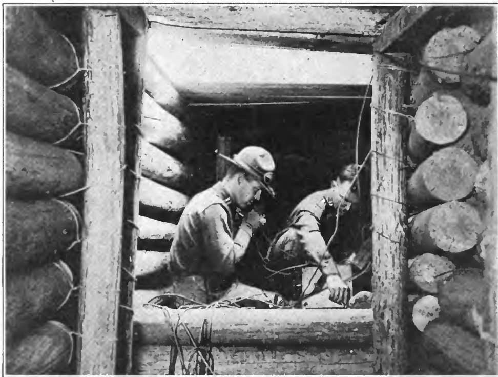
Sample of telephone dug-out in the front line trenches in which the Signal Corps men maintain the lines of communication at all hazards
