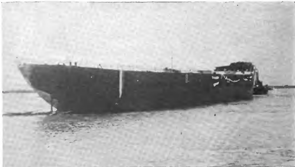
Uncle Sam's new five thousand ton concrete ship Faith, ten times larger than any constructed up to the present time
