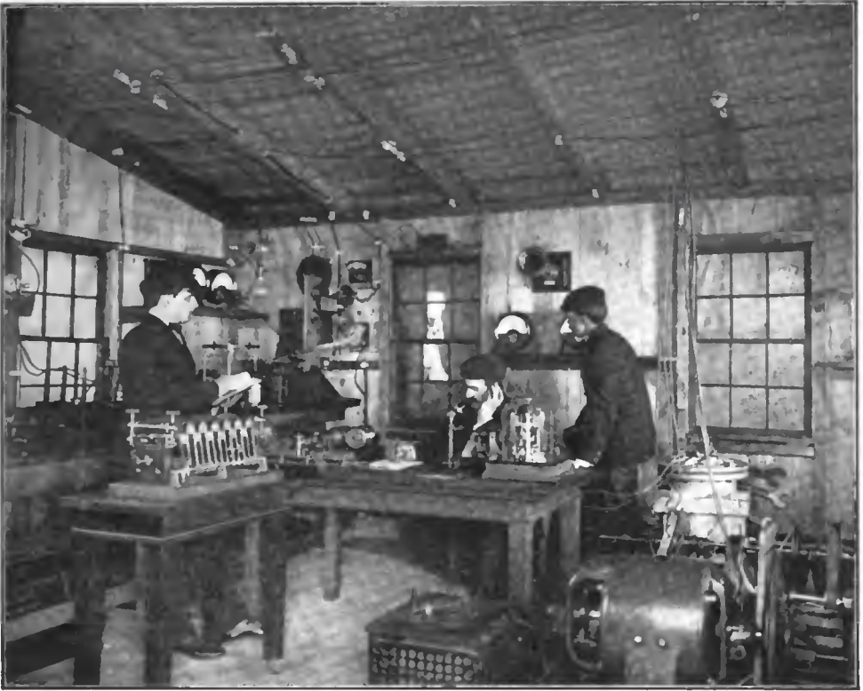
Figure 124—National Electric Signaling Company—Fessenden 2 K.W. radiophone transmitter
