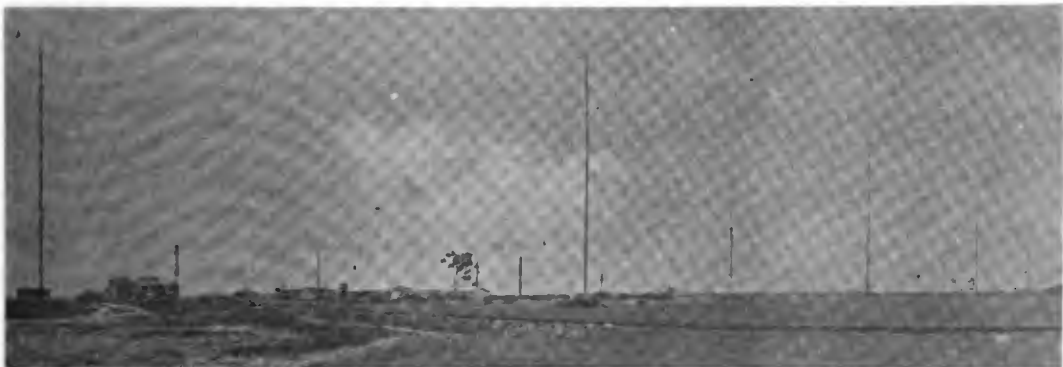
pictured in this photograph, is now employed in the United States-Japan wireless service mast, at the right of the power house (center), and the San Francisco mast at the left
