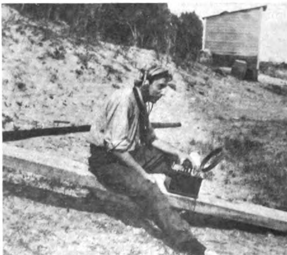
The first wireless station was constructed under great difficulties; it was often necessary to wait two weeks for material and tests had to be made piecemeal
