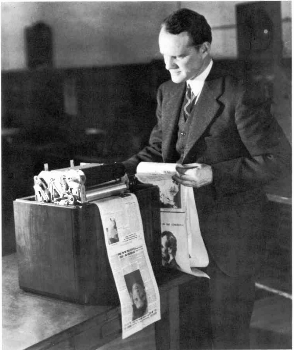
FACSIMILE. During 1937-39 the newspaper-by-radio was considered at the breakthrough point. Above, a 1939 RCA facsimile receiver.
