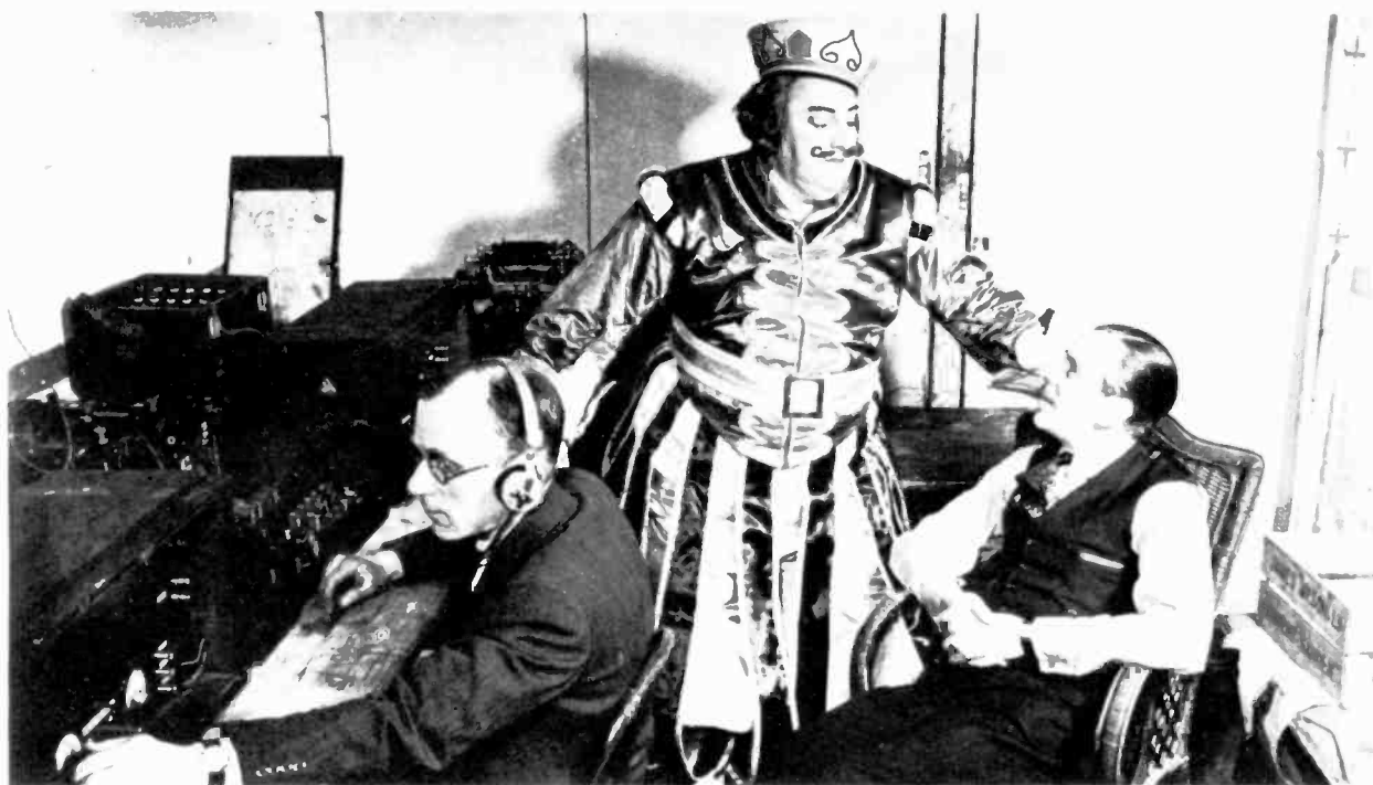
THE BROADCASTING OF PUBLIC PERFORMANCES. SOUND TRANSMITTED THROUGH A MICROPHONE ON THE STAGE TO AN AMPLIFIER BELOW AND THENCE BY TELEPHONE WIRES TO THE BROADCASTING STATION POSSIBLY REMOTE, FOR DISTRIBUTION TO THOUSANDS OF LISTENERS.
