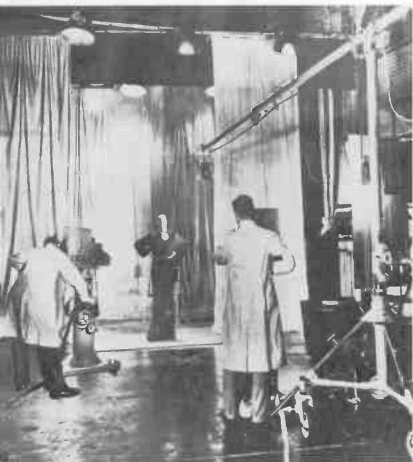
1a Here's Looking at You : Miss Elizabeth Cowell in the announcing position. Note the curtained-off stage, the basic overhead lighting, the microphone suspended from a boom and the Emitron cameras on the unwieldy 'iron man'
