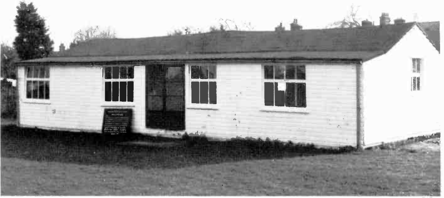
35. From broadcast station to sports hut.
