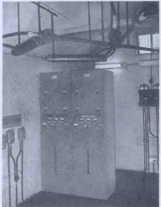
Filter system enabling separate transmitters to feed into a common wide-band aerial
