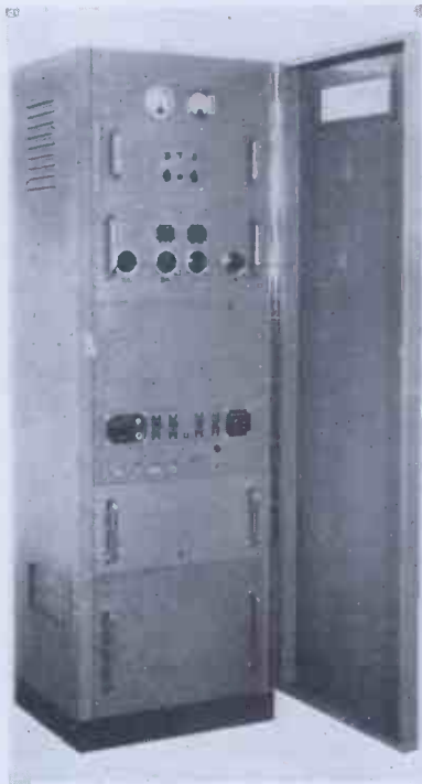
Cooling of the interior of the transmitter is accomplished by a blower, the air intake of which is filtered through a fibre-glass filter.
