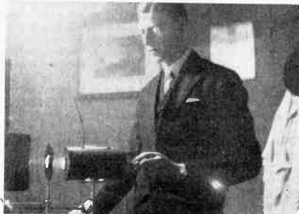
Mr. Ahronheim operating the tungsten lamp of his experimental transmitter.
