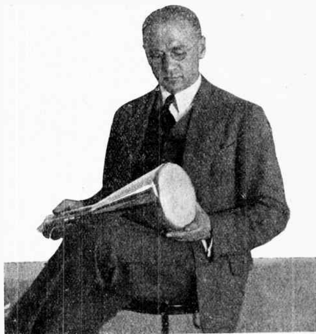
Dr. Zworykin and his new cathode-ray tube, which he calls a "kinescope." The television images appear on the round flat end at right.
