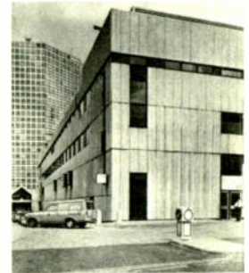
Part of the ATV Centre in Birmingham.
