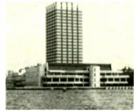
London Weekend's South Bank Television Centre near Waterloo Bridge.
