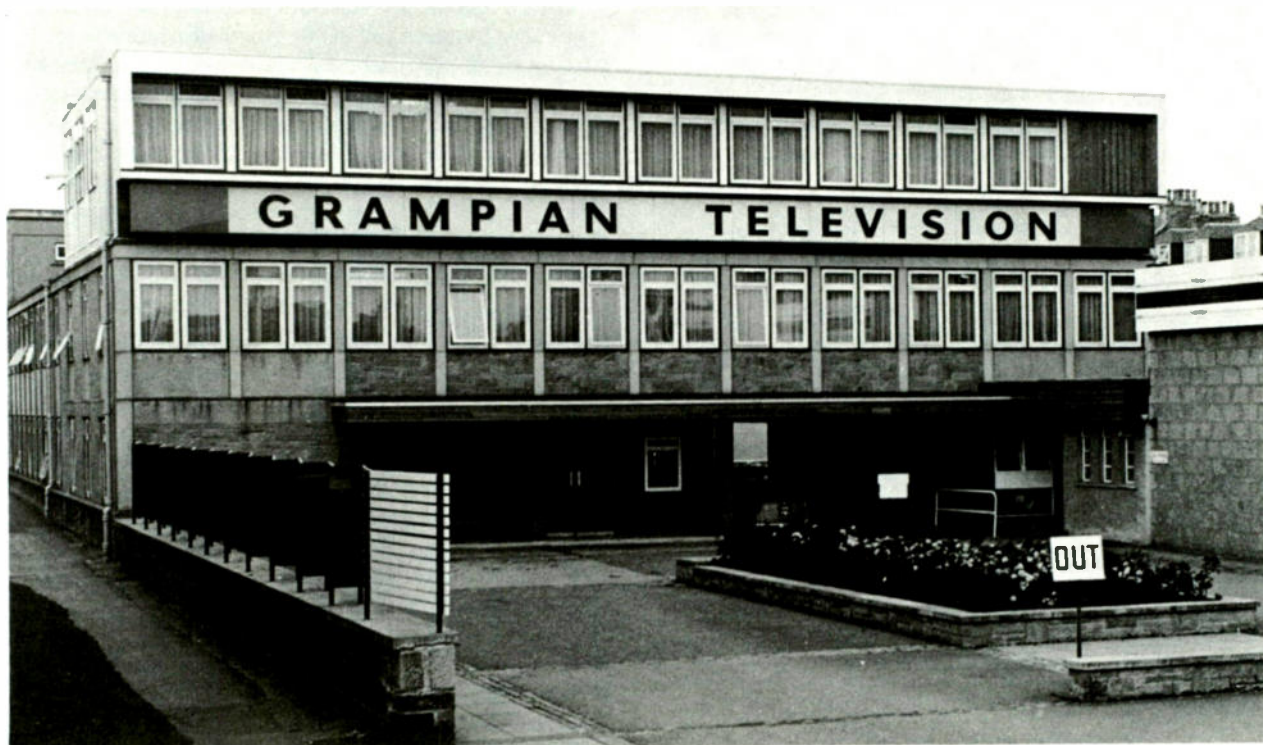
Exterior of Grampian's Aberdeen Studios
