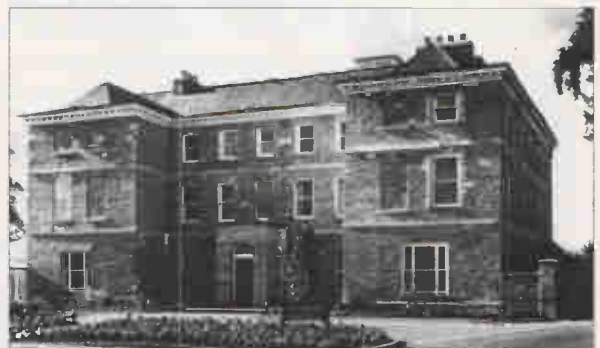
Park House, Hanslope Park.
