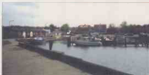
The DX hut (building, on left).
