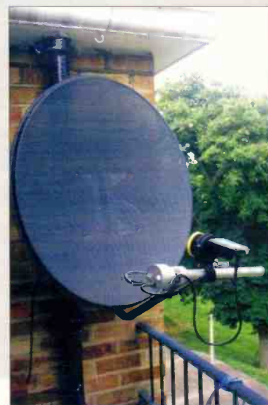
Dean's balcony mounted dish. You can squeeze a dish into most dwellings. Note the multi-sat unit with the LNB clamped to it.
