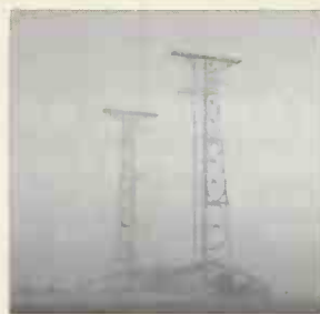
The steerable curtain antenna at Moosbruun.
