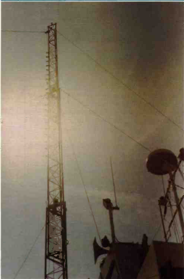
The temporary mast on the MV Yeoman Rose.
