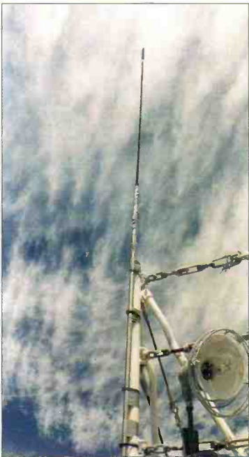
Multiband whip antenna taped to an upper deck stantion.
