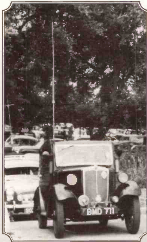
Fig. 3: G2BCX/M arriving at a mobile rally in the Midlands. Valve transceiver for top-bands as in Fig. 1. Antenna 3m long centre-loaded. Probably during 1956.
