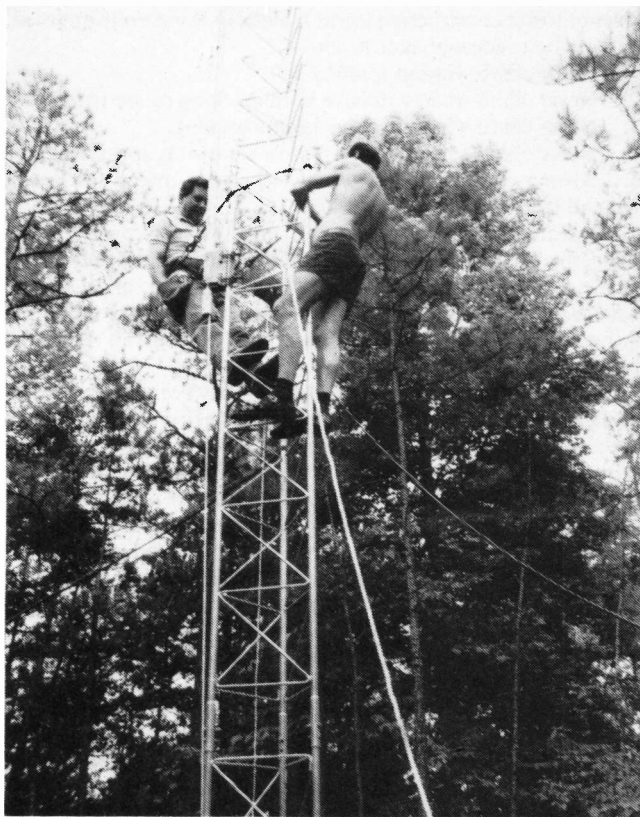
N4TO and G4BUE adding another section of tower.
