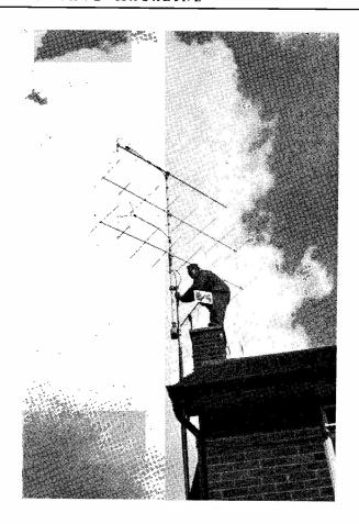
The new beam array for two metres and 70 centimetres at G3COJ, Flackwell Heath, High Wycombe, Bucks.—with G3NBB doing the roof work. (Brian says that somebody has to do the ground work and keep a foot on the ladder!) The two-metre aerial is an 8.8 and the 70 cm. beam a 14-element job.
