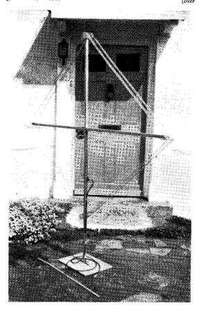
Showing the general construction of the Frame Aerial described in the article, used for transmission as well as reception on Top Band, with very interesting results. On the ground, beside the baseboard, is a 3ft. rule for size comparison. Each section of the winding consists of four turns, with the feed connection at their mid-point (see text and Figs. 1-2).
