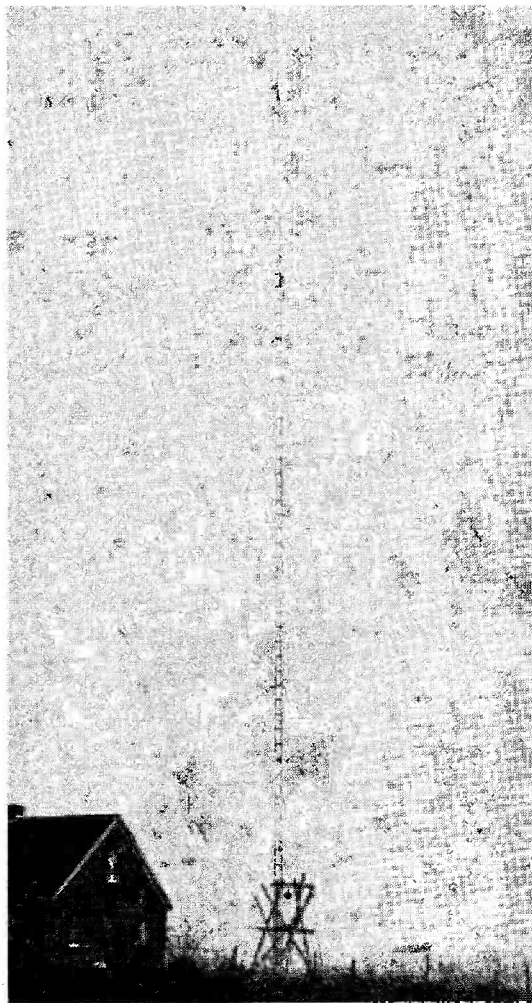
This is the 137-foot vertical mast aerial used on One-Sixty by W8GDQ of Wellington, Ohio.
