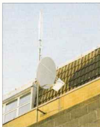
Fig. 5: A typical low power community node.
