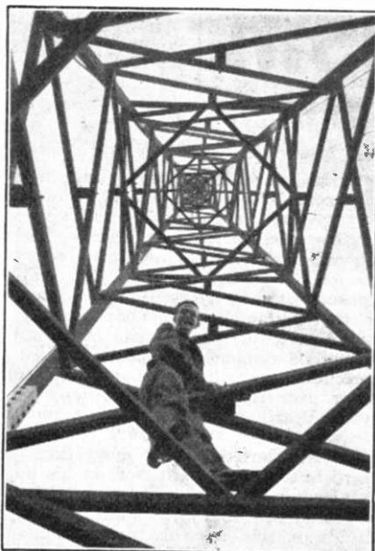
Eddie, of YI2AT, taking a trip up the lattice tower
