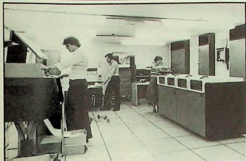
THE WEA computer room—the system was first used at the company's French distribution centre.
