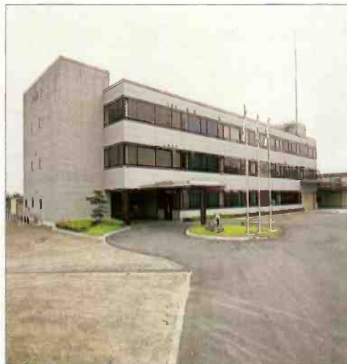
The Yupiteru plant and engineering centre.
