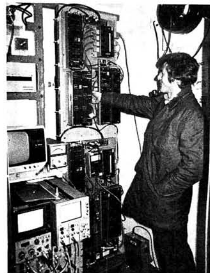
Inside the Hedleyhope relay station
