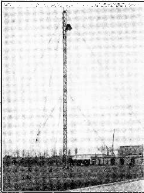
An aluminium test mast erected to half its full height of 200 ft. At the head of the mast the light-alloy erection pole can be seen.
