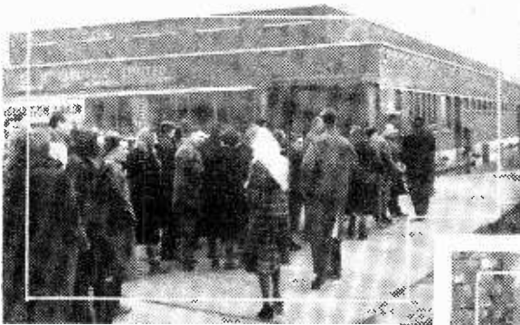
Egen Electric, Ltd., whose Canvey Island factory was surrounded by water as a result of the floods, was soon in production again—the first of the Island's industries to resume work. On the day after the floods took place a skeleton staff of 20 were at work in the factory on essential duties (above). Production recommenced in earnest on Wednesday, February 4th, when power was restored at 11 a.m., and a gradual build-up has taken place as members of the staff have been traced and have reported to work, until at the present time a quarter of the total labour force are again at their duties.
