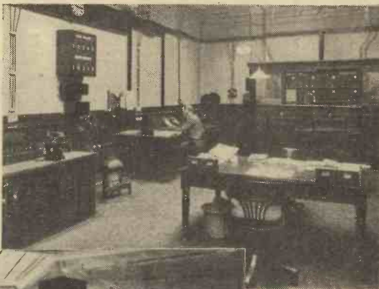
Control Room (2LO) prior to 1931, showing the Simultaneous Broadcasting Board and Control Desk in background.
