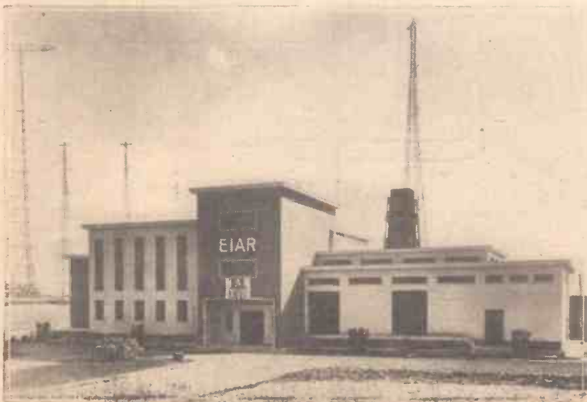
A front view of Italy's new broadcasting station recently opened by Signor Mussolini, at Prato Smeraldo, five miles to the south of Rome. It is claimed that this station, known as the Imperial Radio Centre, is the most powerful and best equipped in the world.
